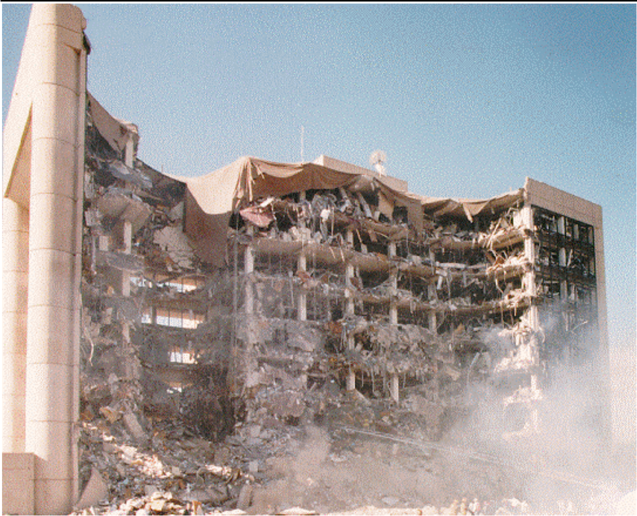
Murrah Federal Building
